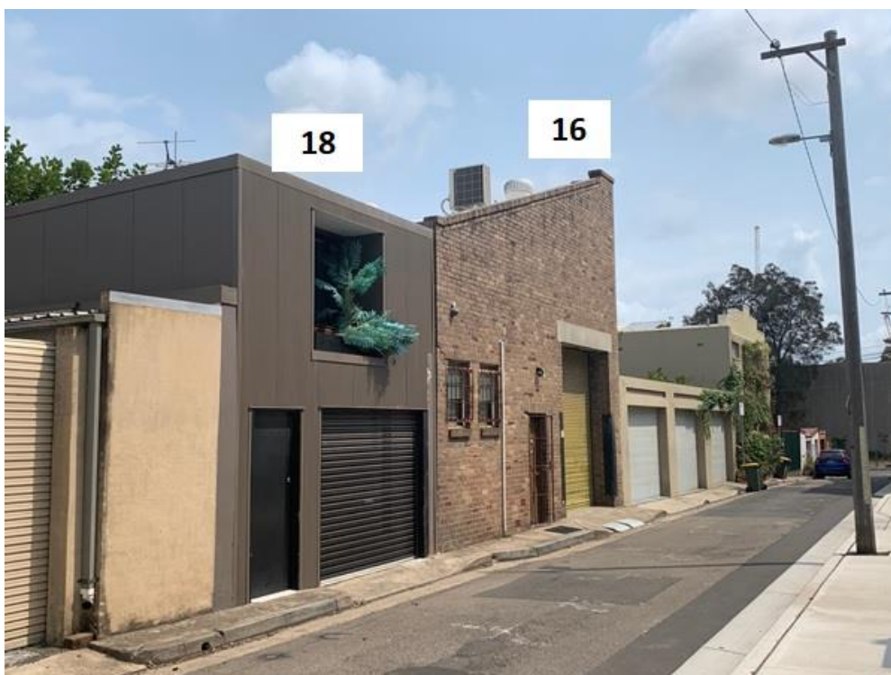
Figure 32: Salisbury Lane frontages of two-storey laneway building at no. 18 and warehouse at no. 16 Princess Avenue.
