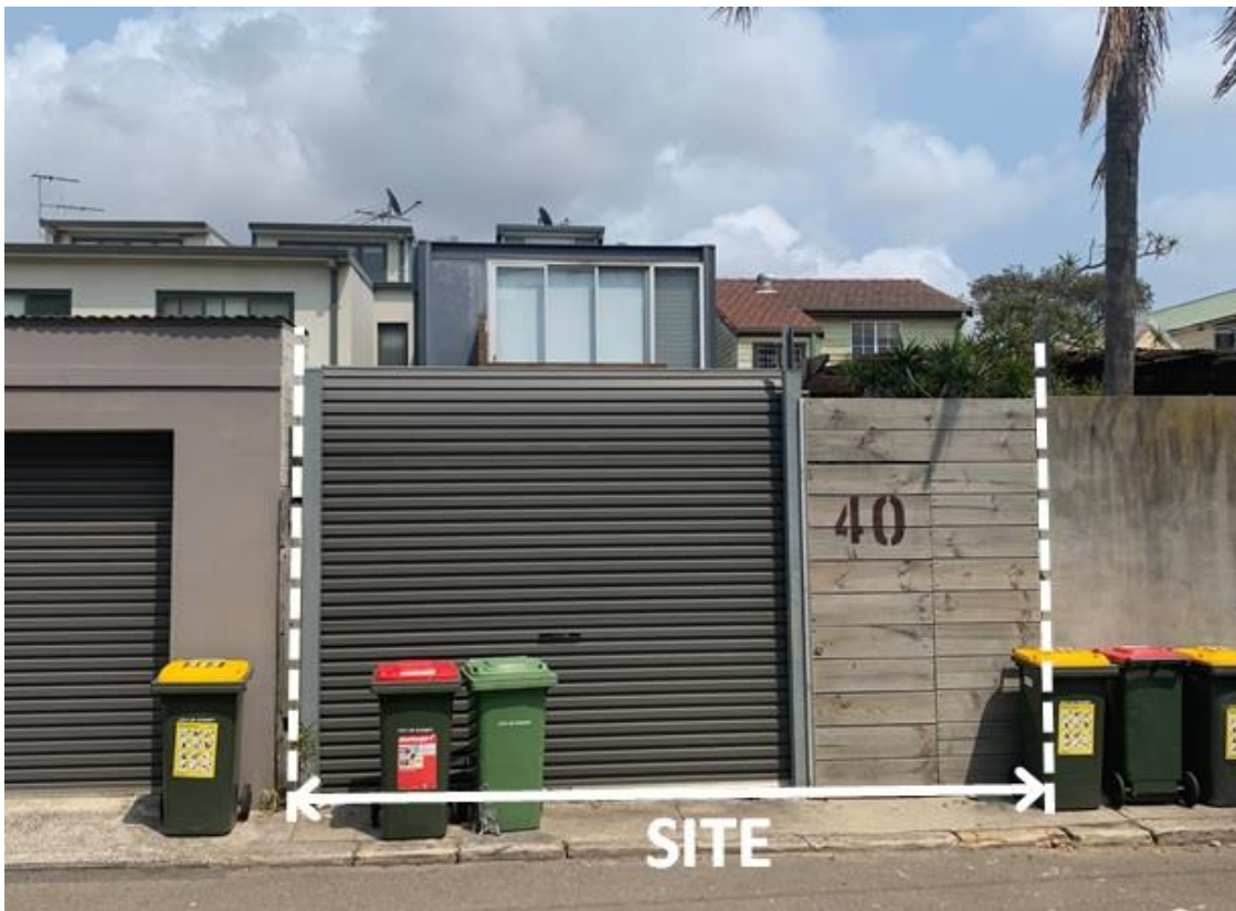
Figure 3: Existing roller door and gate to site's Salisbury Lane frontage.
